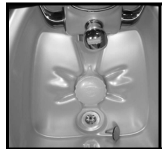
Drain plunger removed
